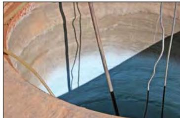
The bright, highly reflective blue epoxy coating nears the top of a manhole.
